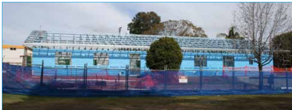
South Grafton Public School Library under construction, August 2010
